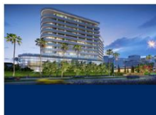
For the refinancing of senior debt on the Beverly Hilton Hotel and Waldorf Astoria Beverly Hills, California USA
